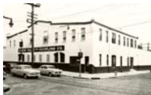
Warehouse and shipping building at 2nd and Columbia in Philadelphia
